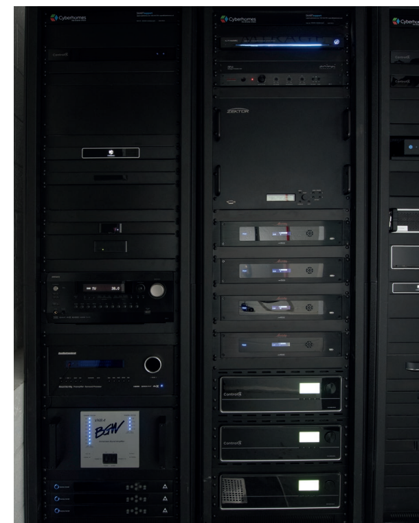
All equipment is installed in dedicated AV racks in the plant room, minimising the technology's impact on the home's interior design
